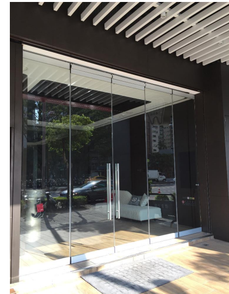
Movable double swing & sliding panel with hydraulic control
