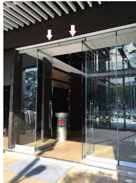
Movable double swing & sliding panel with hydraulic control
