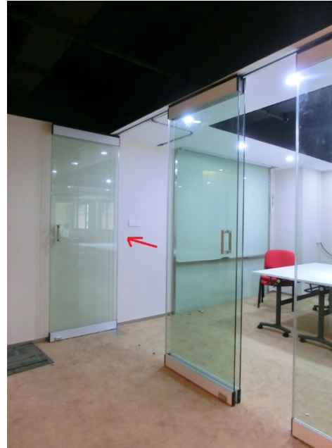
Movable double swing & sliding panel with hydraulic control
