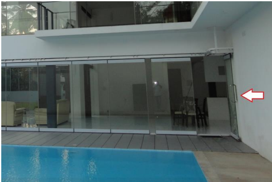
Fixed Double swing panel with hydraulic control
